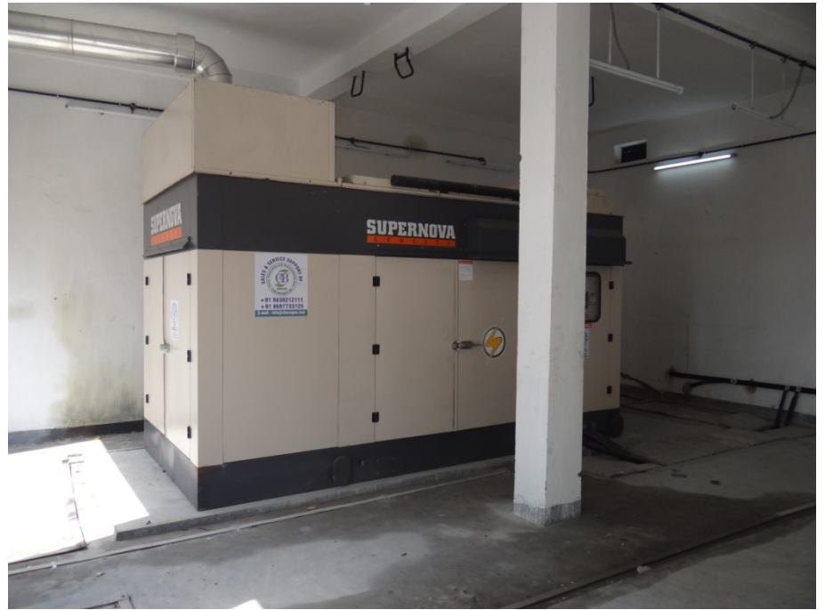
380KVA SUPERNOVA VOLVO PENTA DG SET AT AMBUJA CGL HOTEL
