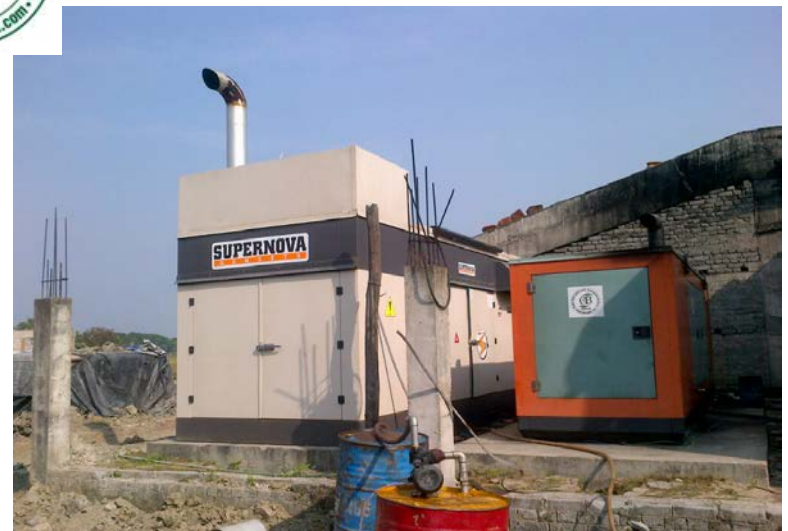
600KVA VOLVO PENTA & 160KVA COOPER AT VEDIC VILAGE
