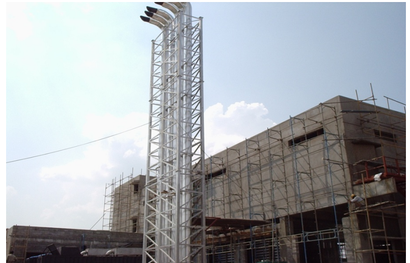
STRUCTURAL SUPPORTED DG EXHAUST LINE
