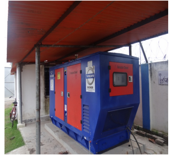
62.5KVA VOLVO EICHER DG SET AT TTSP
