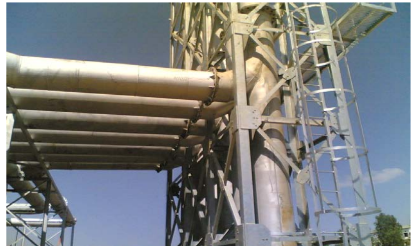
DG EXHAUST HORSE SHOE JOINTS
