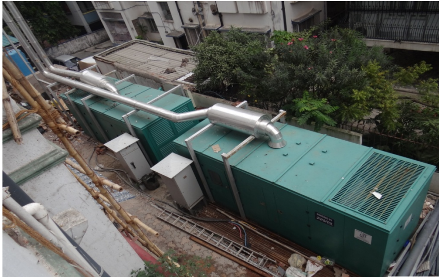
2X380KVA DG INSTALLATION & SOUND PROOF ENCLOSURE & OUTDOOR PANEL AT AMRI SALT LAKE
