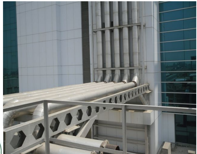
INSULATED DG EXHAUST LINE
