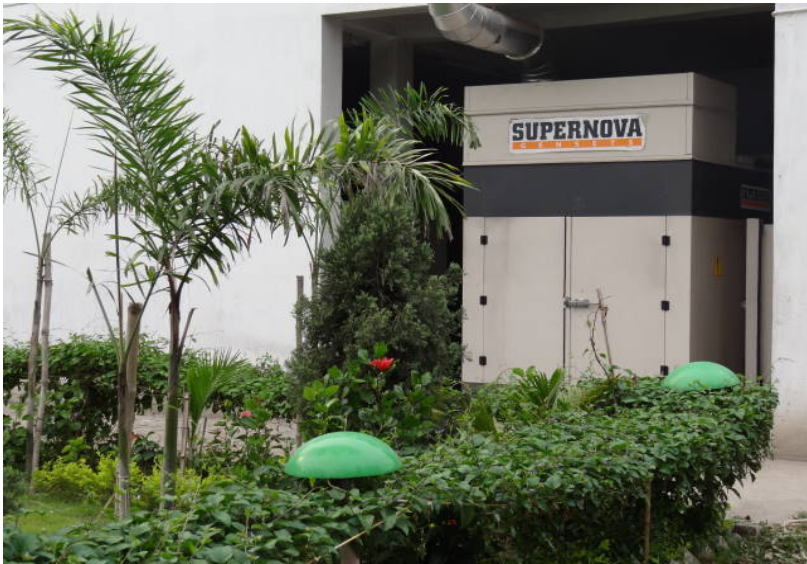
450KVA VOLVO PENTA DG AT PC COLOR SOFT
