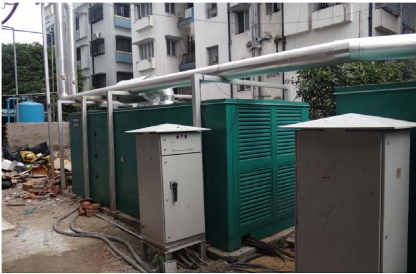
2X380KVA DG INSTALLATION & SOUND PROOF ENCLOSURE & OUTDOOR PANEL AT AMRI SALT LAKE.
