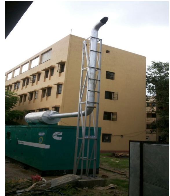
500KVA CUMMINS DG INSTALLATION AT AMBUJA RAICHAK
