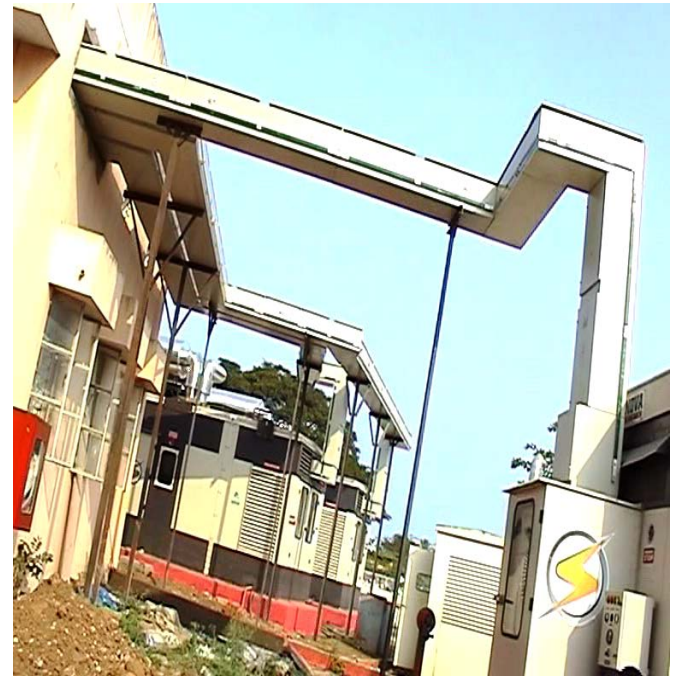
1250KVA SUPERNOVA PERKINS DG WITH BUS DUCT
