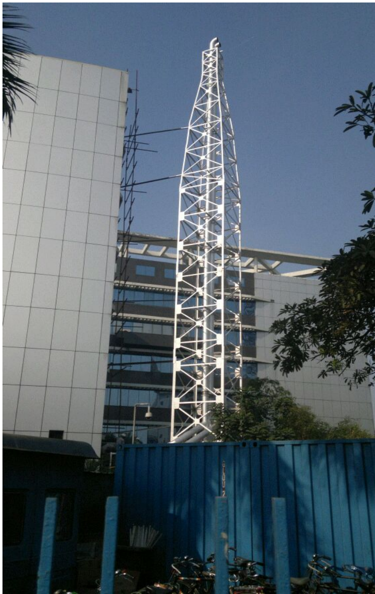
DG EXHAUST TOWER FOR 750KVA & 1250KVA AT CTS KOLKATA
