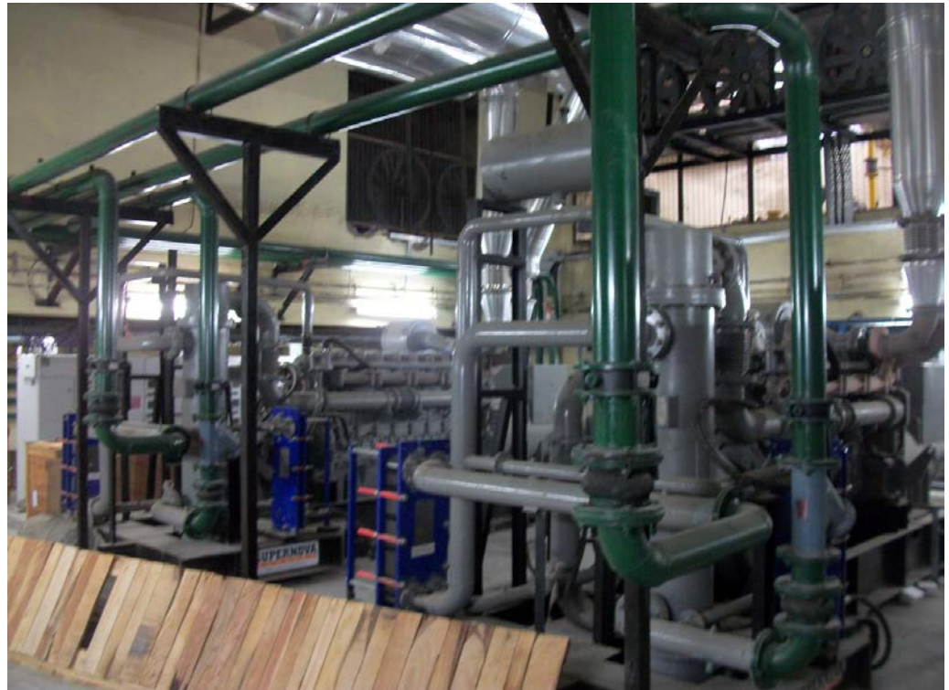
2X1700KVA HE COOLED SUPERNOVA PERKINS DG SET
