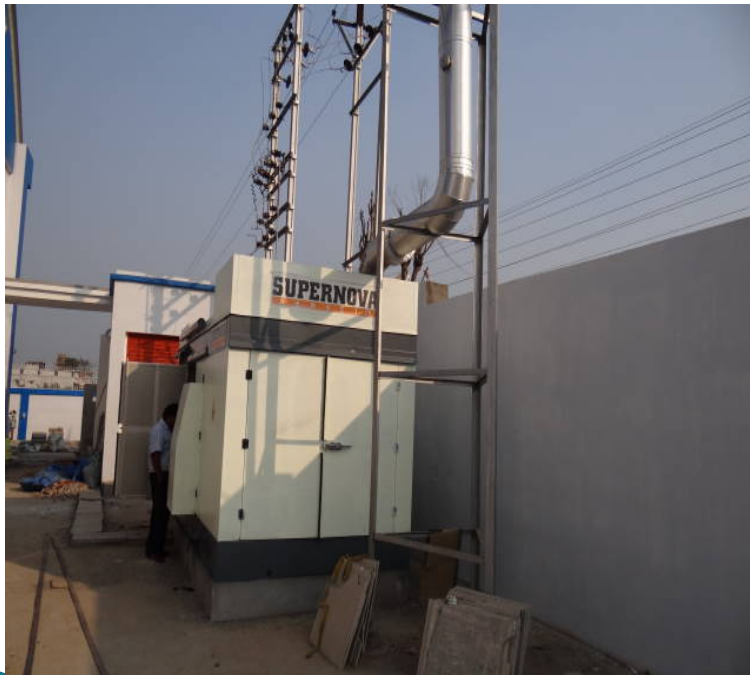
250KVA SUPERNOVA VOLVO PENTA AT AFFAPL.
