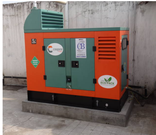
25KVA COOPER DG AT SWAMAK INT. JUNGLEPUR
