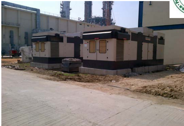
2X1250 KVA SUPERNOVA PERKINS DG & 180KVA AT BERGER PAINTS
